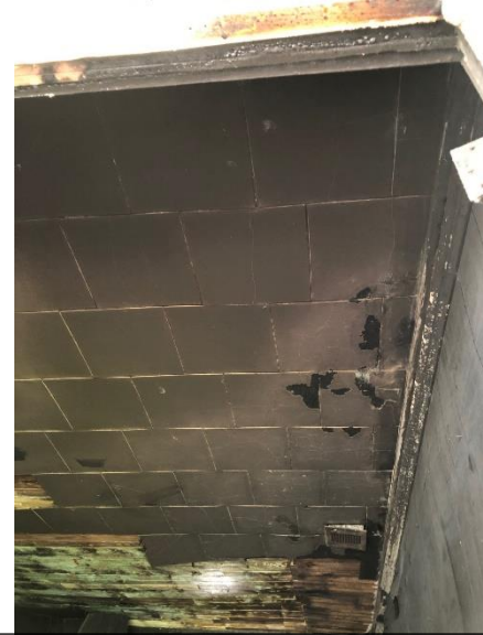
HA 1 – Brown surfaced ceiling tiles
